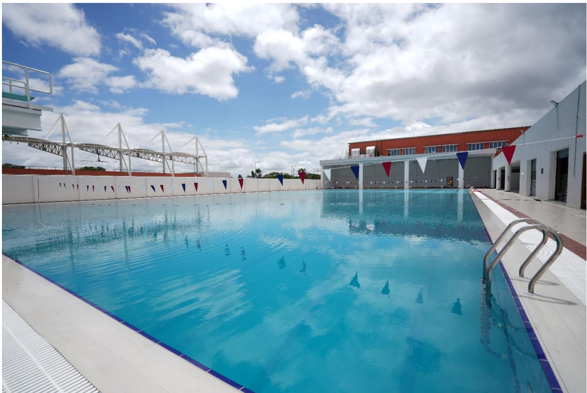
Olympic Swimming Pool
